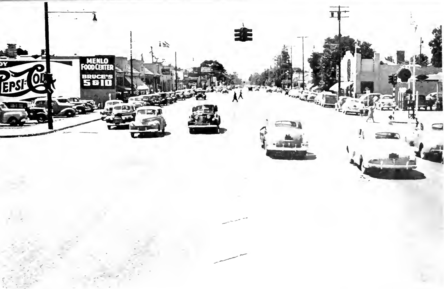
Top, improved section of U. S. 101 showing channelized division strip approaching Atherton. Below, weekend avenue through Menlo Park.
